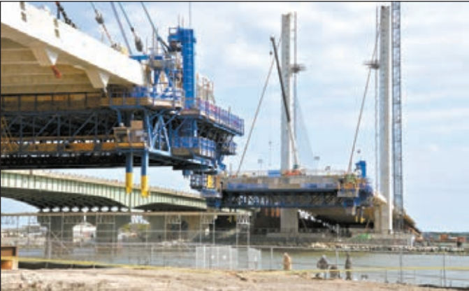
RON MACARTHUR PHOTO Three-fourths of the blue cable stays are in place as the bridge is under construction.
