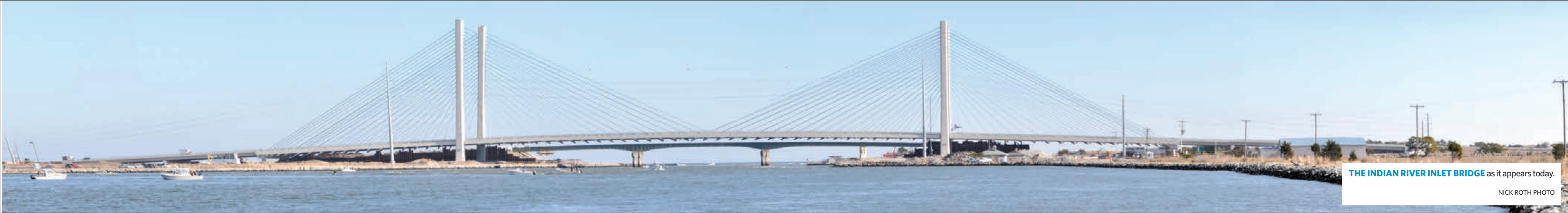
RON MACARTHUR PHOTO Three-fourths of the blue cable stays are in place as the bridge is under construction.
