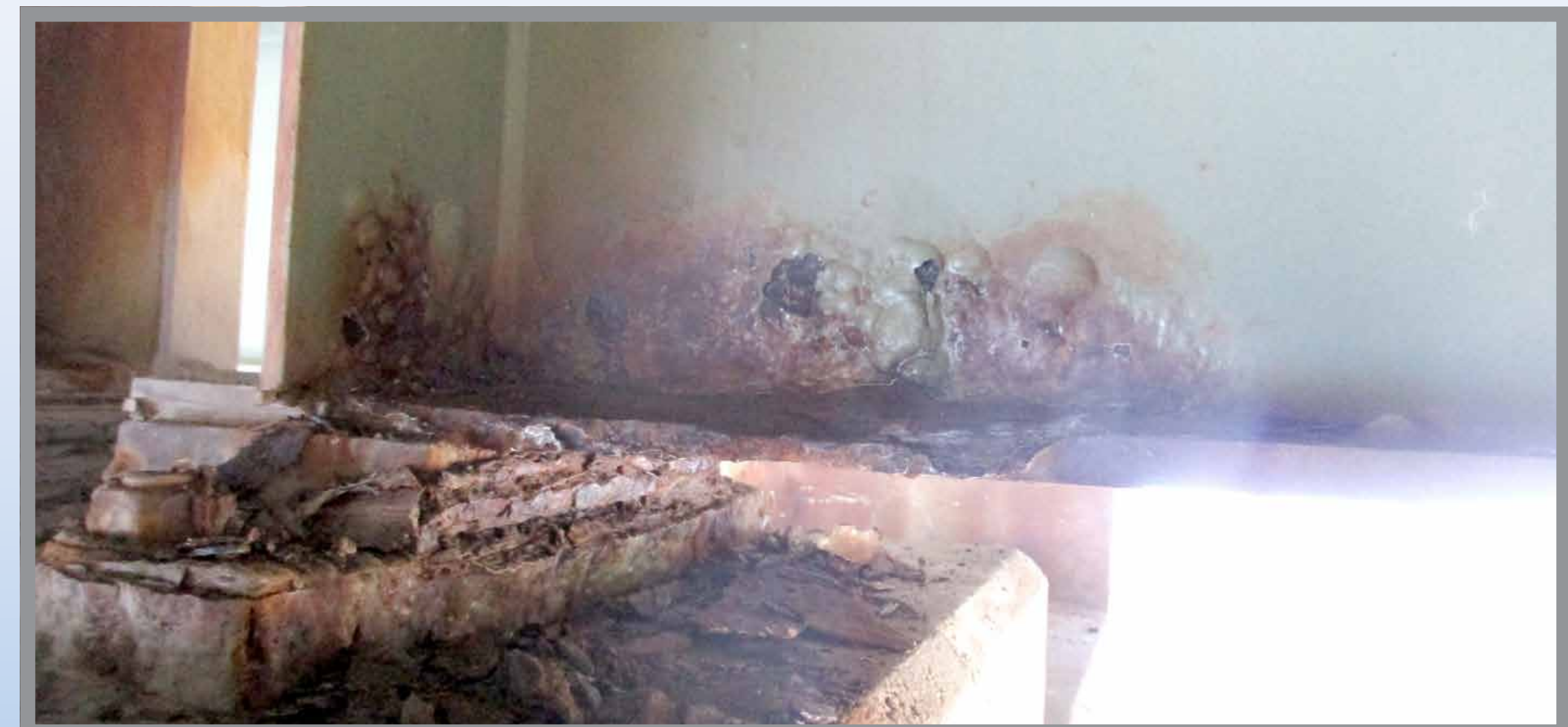
Typical deterioration of the beam ends and bearings
