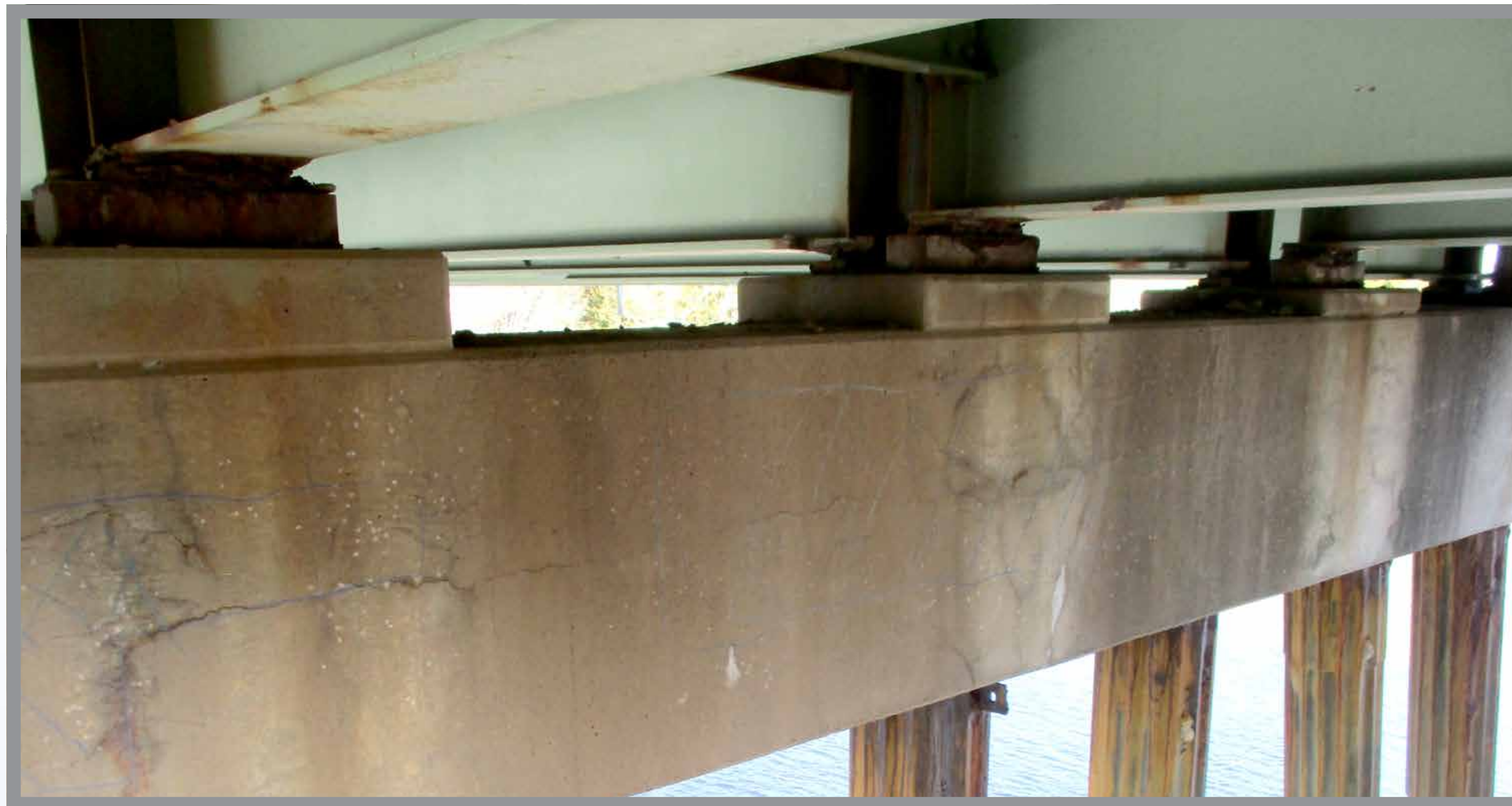
Concrete deterioration along bridge pier
