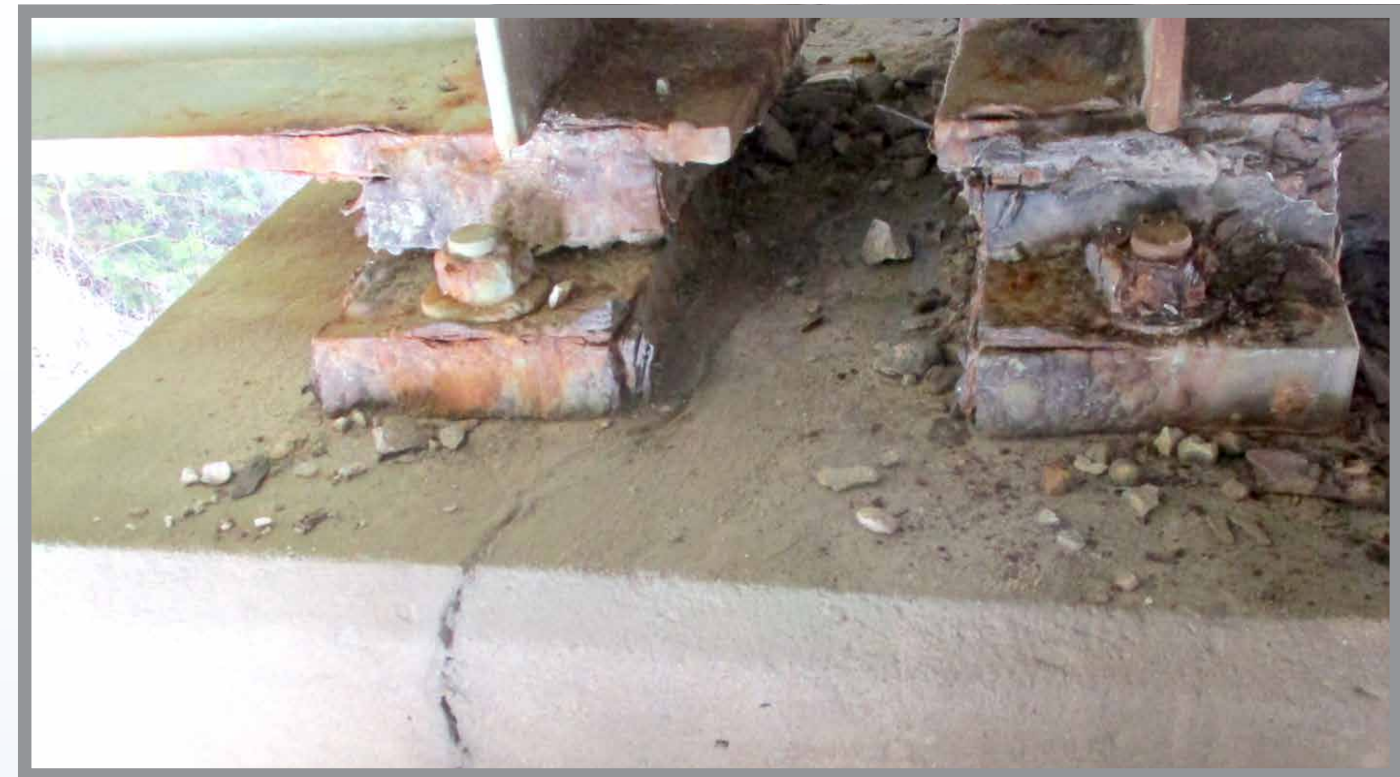
Deterioration of steel bridge bearings and supporting concrete
