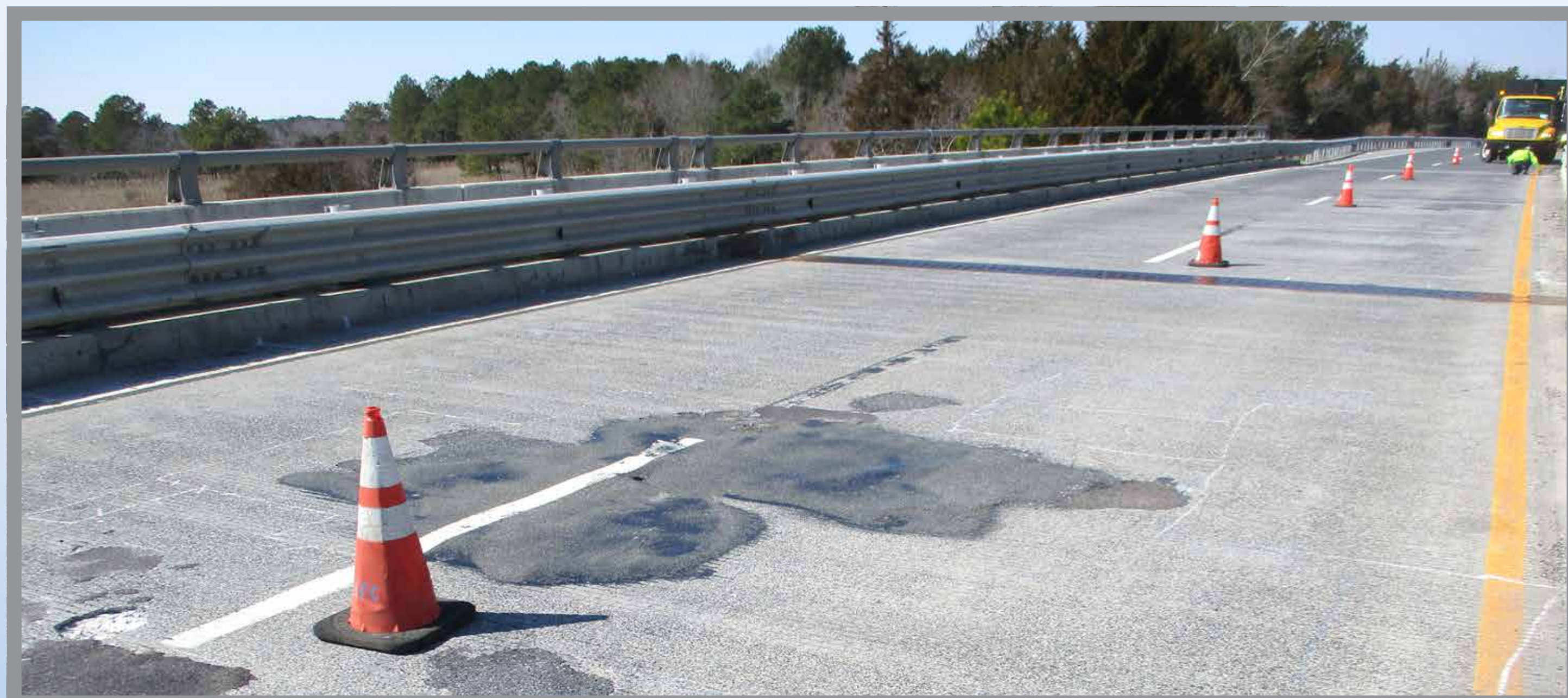
Deterioration of southbound bridge deck
