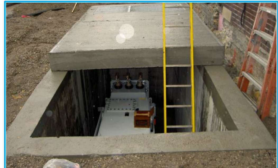
U.G. TRANSFORMER VAULT EXAMPLES
